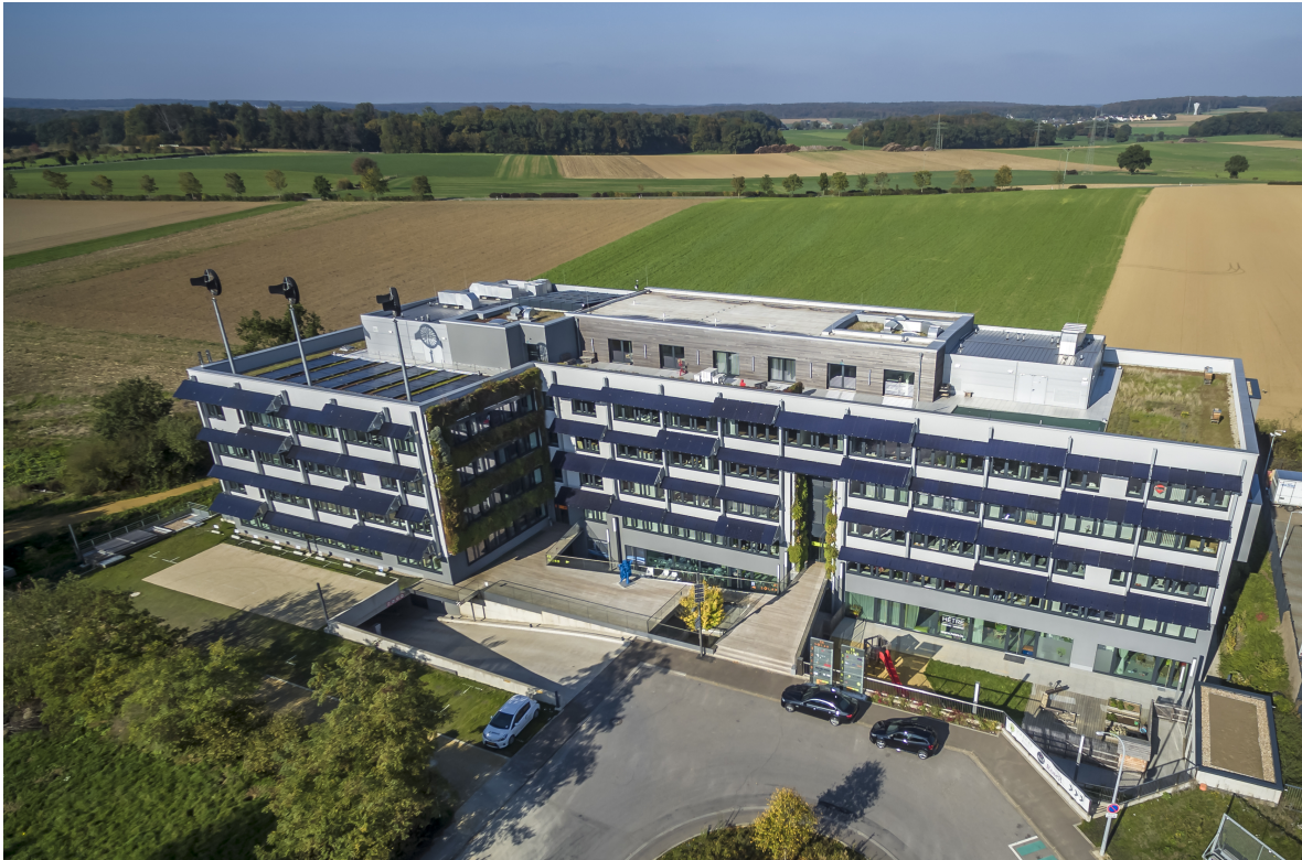
Figure 1: Aerial photograph of Solarwind and its surroundings. The PV panel shading on the south façade, green roof, green façade and solar thermal collectors are clearly visible. At the east façade one of the boxes is visible. Courtesy of PROgroup.
